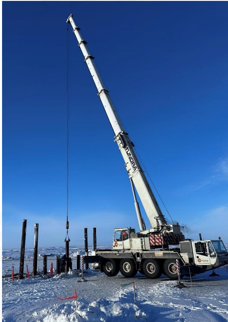
Bridge Pile Installation
