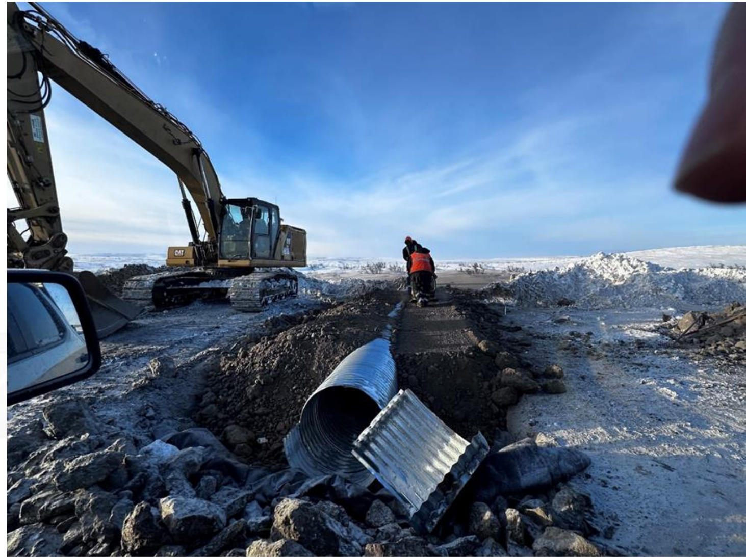
Culvert Installation
