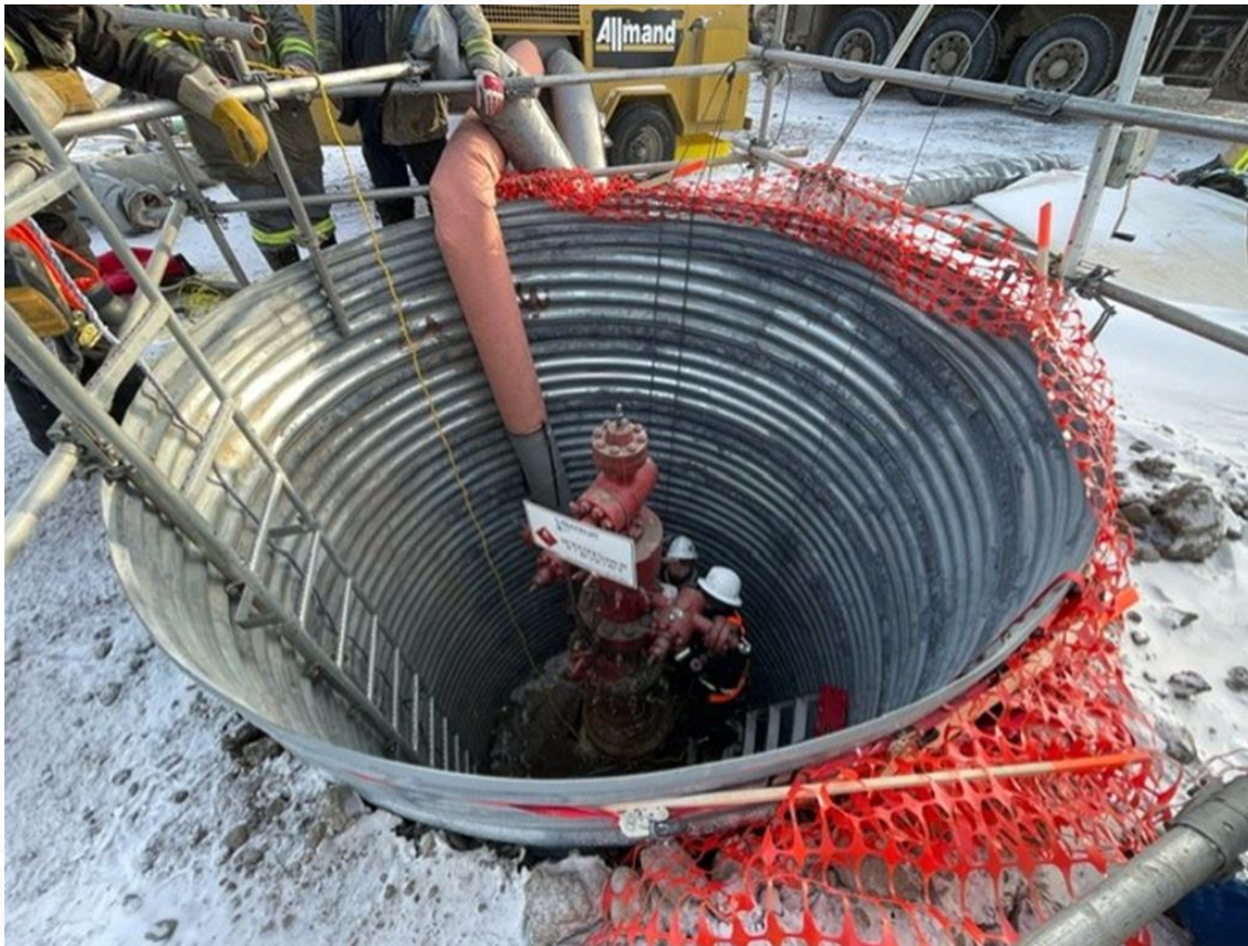
Preparing to Remove the M-18 Wellhead
