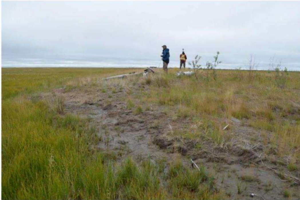
Photograph 4. Close-up view of sump cap erosion along sump perimeter, Langley K-30 sump. Taken August 2018.
