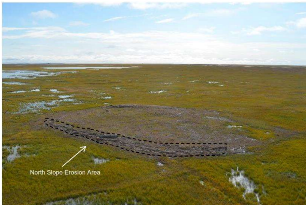
Photograph 3. Example of sump cap erosion along sump perimeter, Langley K-30 sump. Taken August 2018.
