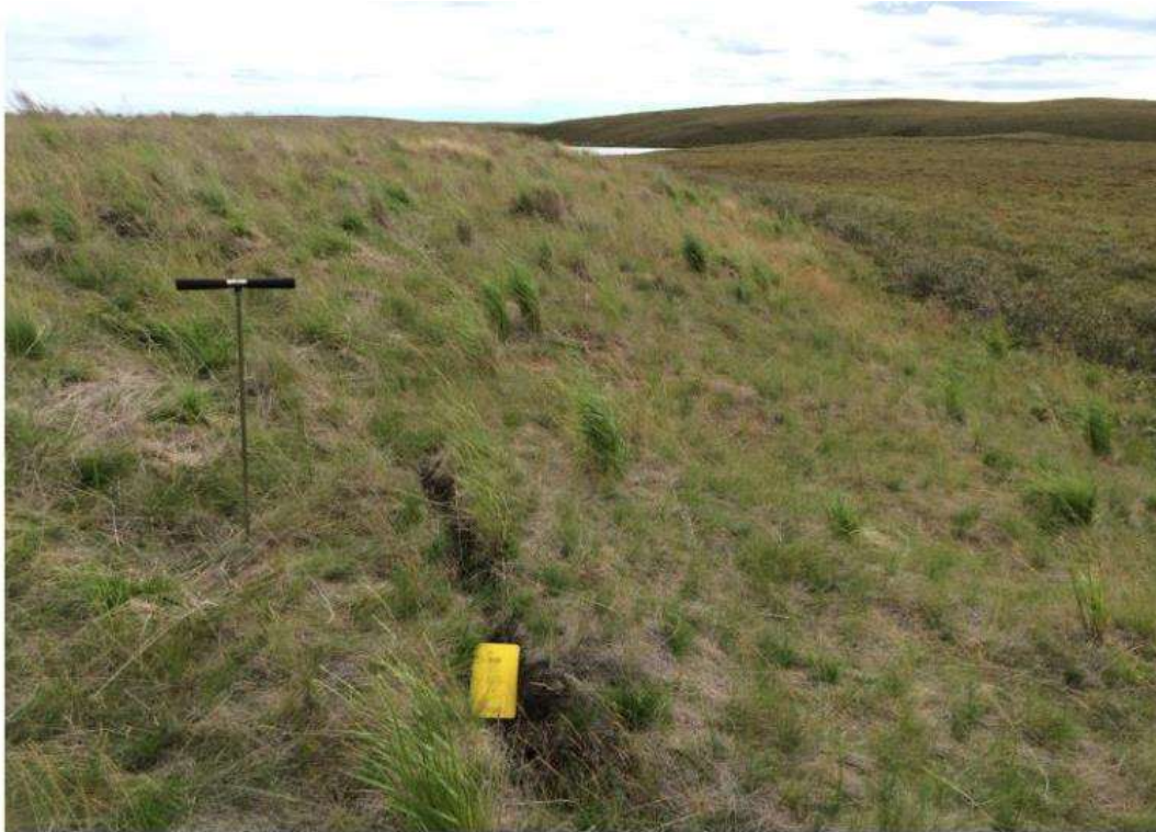
Photograph 6. Example of tension cracking along perimeter of sump cap, Umiak N-05 sump. Taken August 2016.
