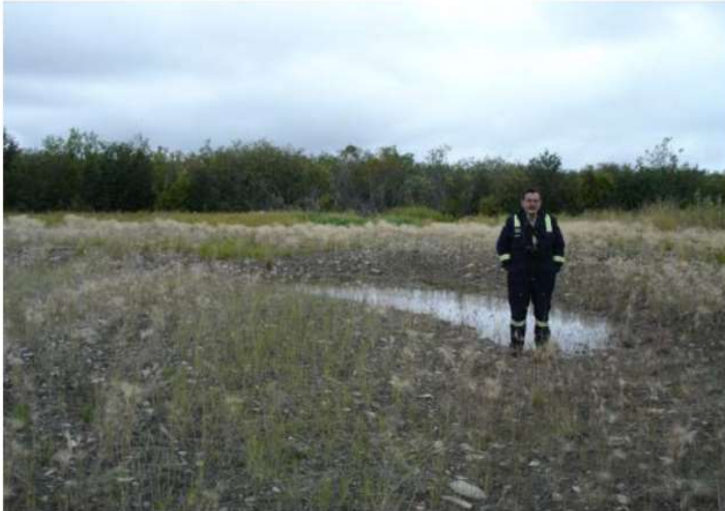
Photograph 2. Example of subsidence of 30 to 50 cm along corner of sump cap, Itiginkpac F-29 sump. Taken August 2013.
