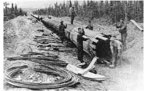
A wood-stave pipe used to carry water to Klondike placer mines.
