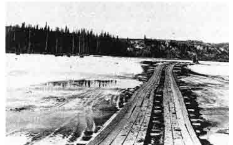
Plank road on the ice across the Peace River, part of the Alaska Highway, 1942.
