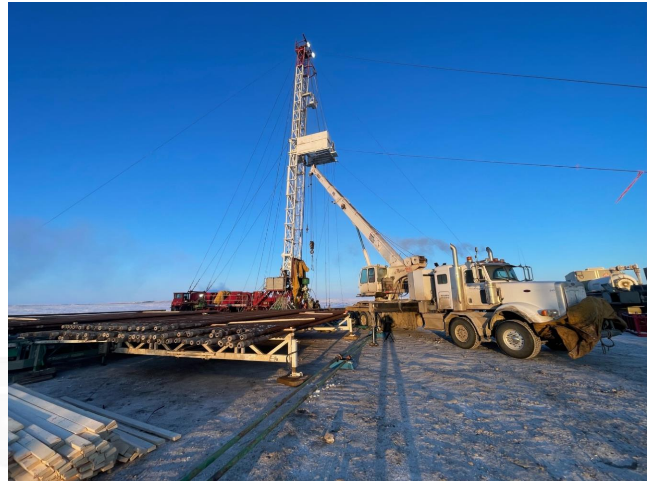
Rig Standing with Work String in Position March 7, 2024
