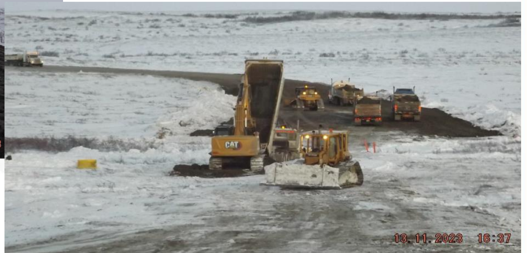
Material Spreading, SW Side of Creek
