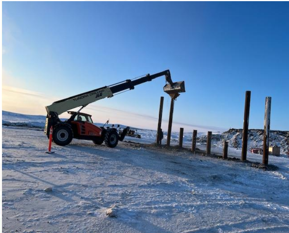
Preparing for girders
