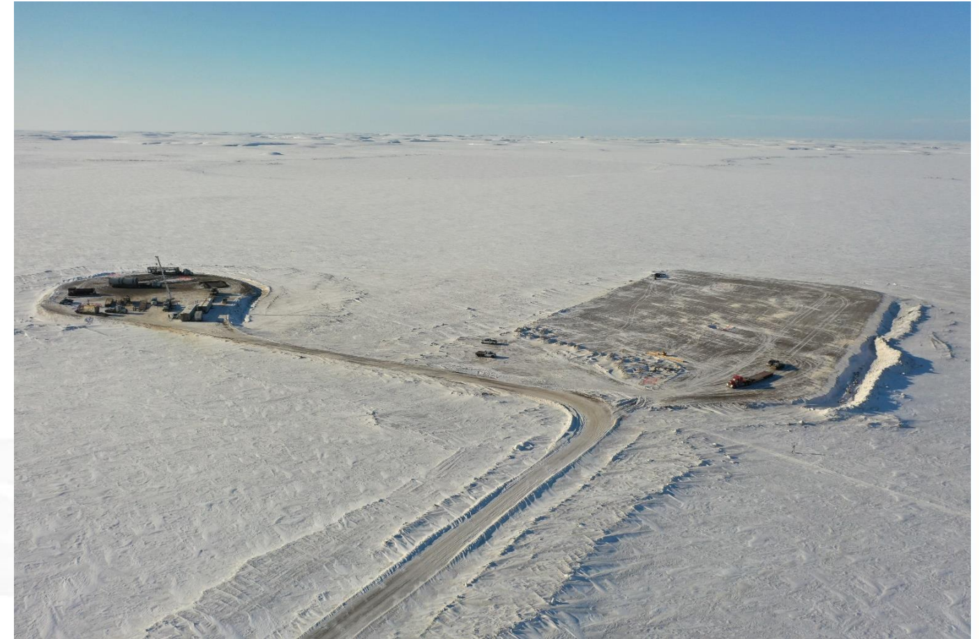
Well Pad/Sump Cap and Energy Centre Pad
