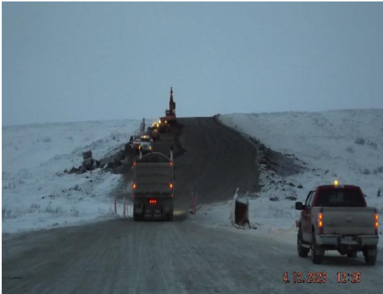
Road construction at hill looking west
