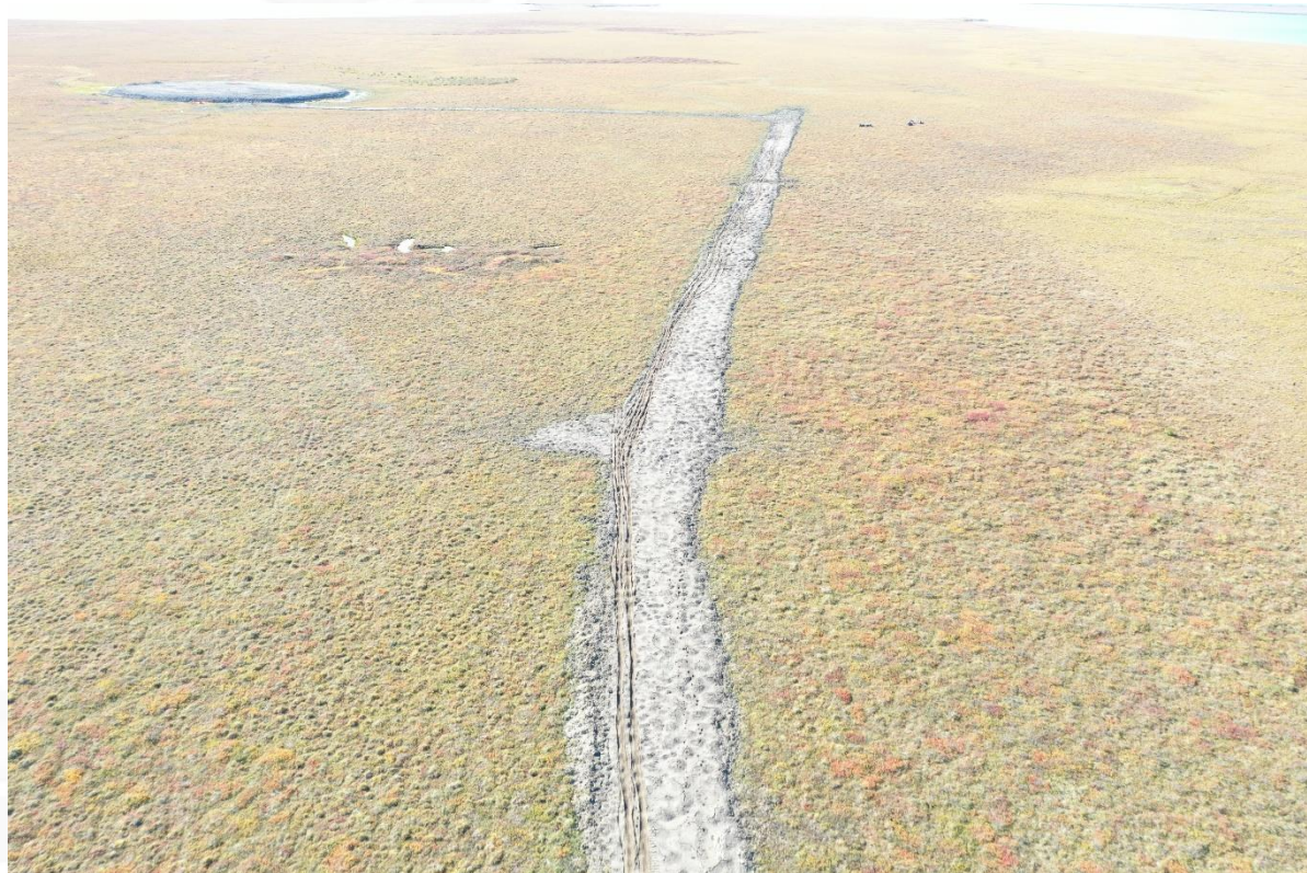
Access Trail Approaching Future Energy Facility Site and M-18 Needed for Access to M-18 and for Sump Remediation
