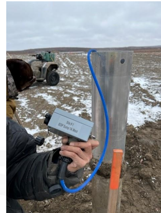
Sump Cap: Ground Temperature Cable
