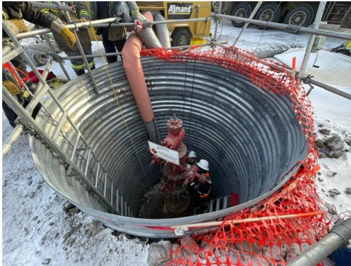
Preparing to Remove the M-18 Wellhead
