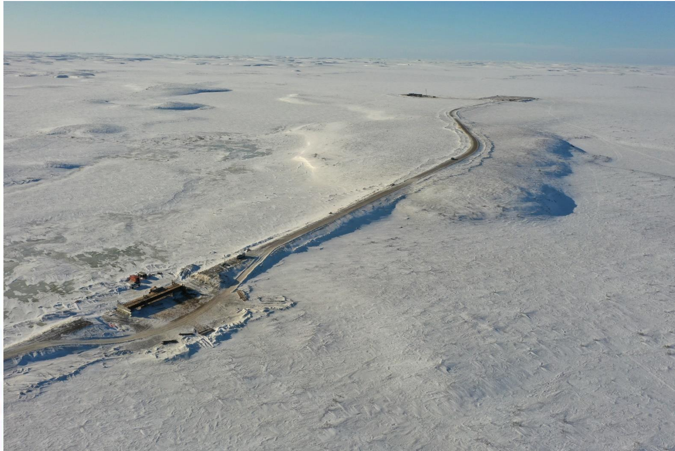
Bridge and Road to Pads
