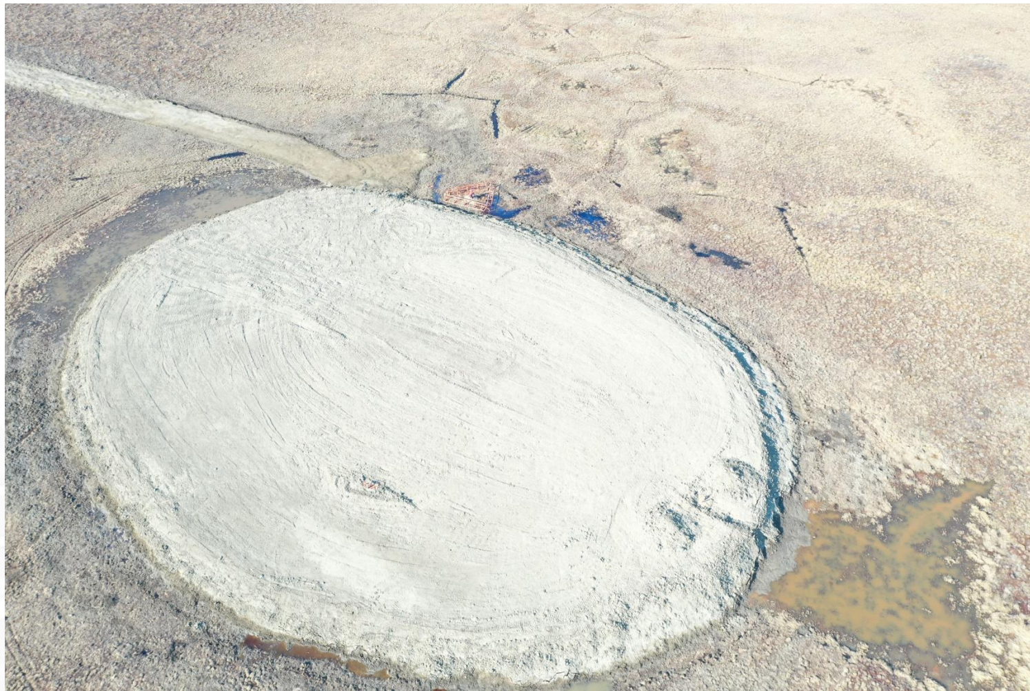
Remediated M-18 Drilling Waste Sump
