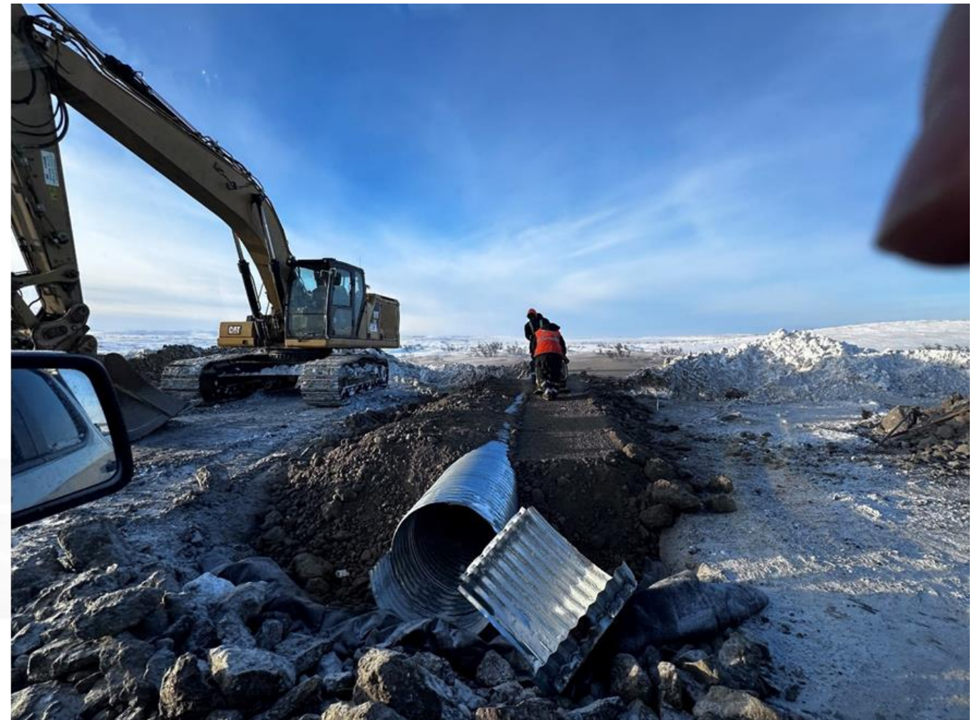
Culvert Installation
