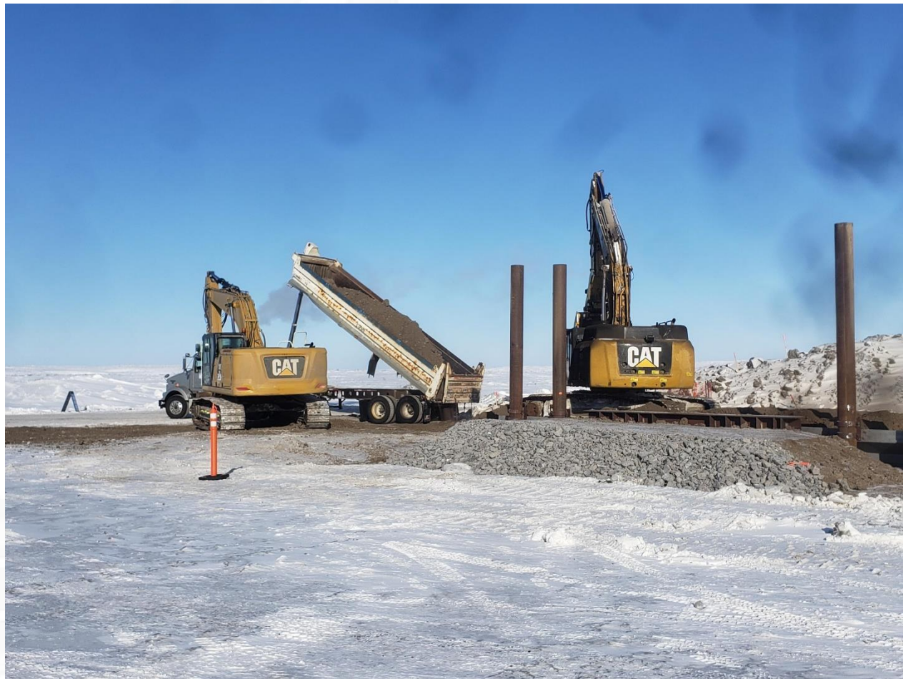
Placement of material at abutments
