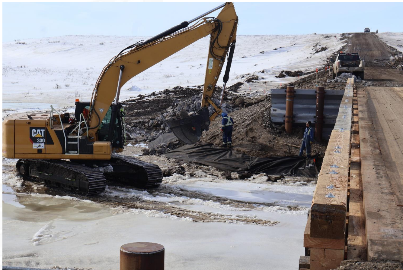
Placing geotextile and riprap
