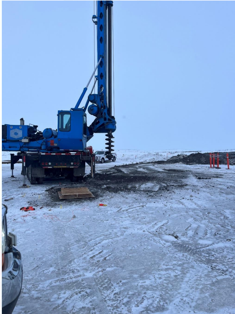
Placing Ad Freeze Piles – February 2024
