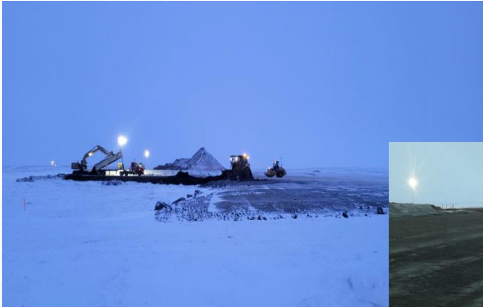
Energy Facility Pad Construction
