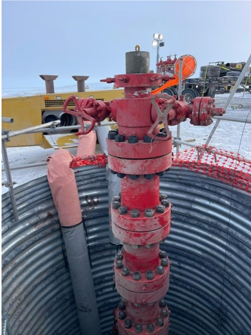
Wellhead Extension – March 3, 2024
