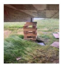
Unstable blocks should be dug out to flat, solid ground and set on compacted crushed rock.
